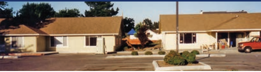
Moorpark buildings B & C
