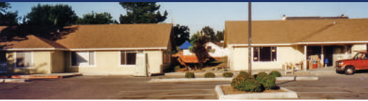
Moorpark buildings B & C
