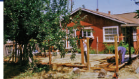
Building Moorpark Infant Center
